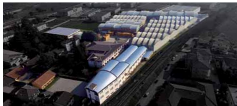
SCAB sede/headquarters - Coccaglio (BS) Italy
