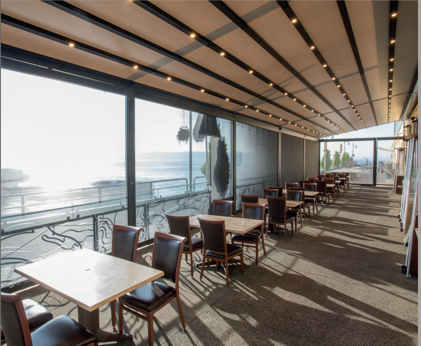
Genius A2C installed by Seattle Shade & Awning
